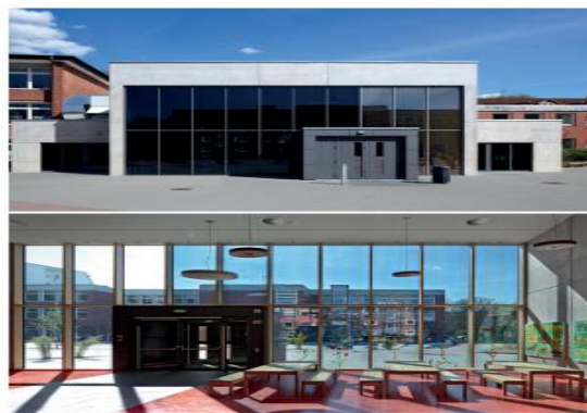
Figure 10. Façade en vitrage intelligent (Source : Smart Films International, Electrochromic glass)
